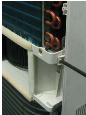
Screws on front bottom of the unit.
